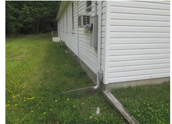
Downspouts on the northern side of the building can be disconnected into a bioretention system to capture, treat, and infiltrate rooftop runoff. A preliminary soil assessment suggests that the soils have suitable drainage characteristics for green infrastructure.
