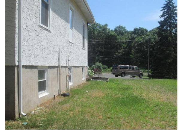
Downspouts along the eastern and western sides of the building can be disconnected into bioretention systems to capture, treat, and infiltrate rooftop runoff. Porous asphalt can replace existing parking spaces to allow water to infiltrate. A preliminary soil assessment suggests that the soils have suitable drainage characteristics for green infrastructure.
