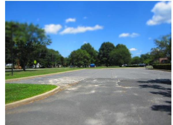
Parking lot runoff can be captured by installing porous asphalt in four strips of parking spaces to help manage stormwater. A bioretention can be installed in the corner of the eastern parking lot to capture, treat, and infiltrate parking lot runoff. A preliminary soil assessment suggests that the soils have suitable drainage characteristics for green infrastructure.
