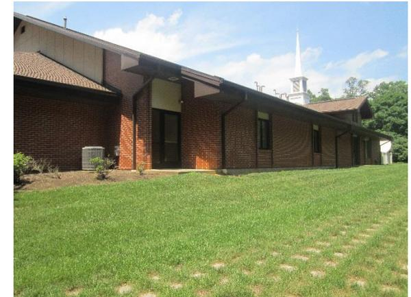
Downspouts on the eastern side of the building can be disconnected into a bioretention system to manage rooftop runoff. Porous asphalt can be used to replace two strips of parking spaces to allow parking lot runoff to infiltrate. A preliminary soil assessment suggests that the soils have suitable drainage characteristics for green infrastructure.
