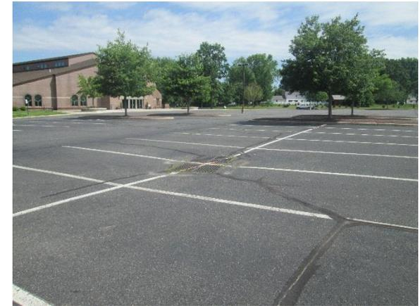
Parking spaces can be replaced with pervious pavement to infiltrate runoff. A preliminary soil assessment suggests that more soil testing would be required before determining the soil's suitability for green infrastructure.
